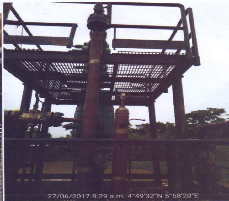
D: SPILL POINT AFTER REPAIRS
